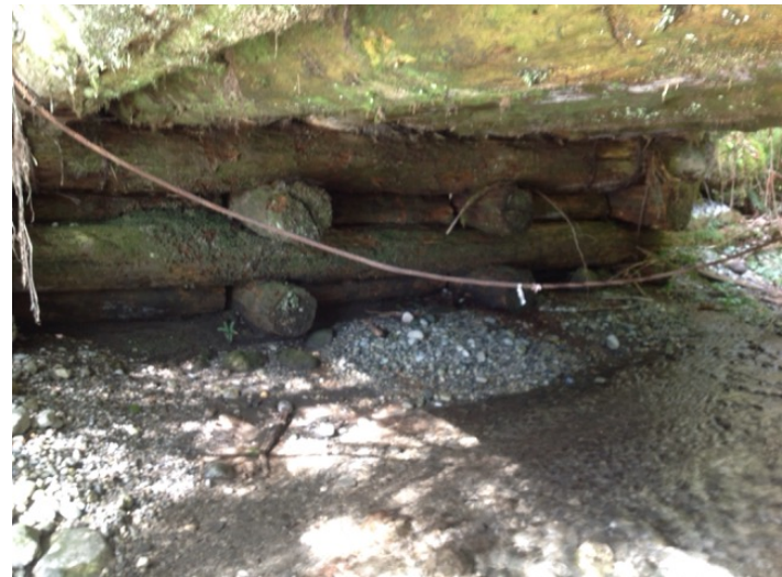
Right Bank Abutment when facing downstream
