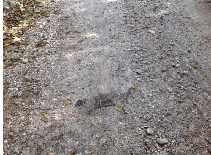
top log stringer exposed
