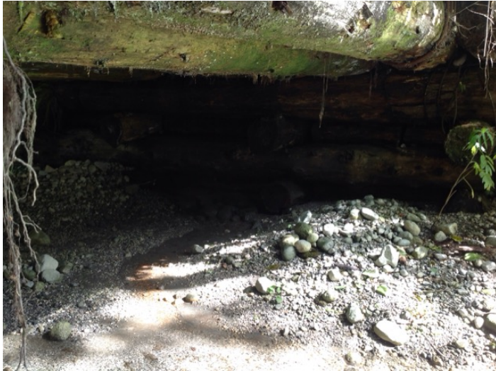
Left Bank Abutment when facing downstream
